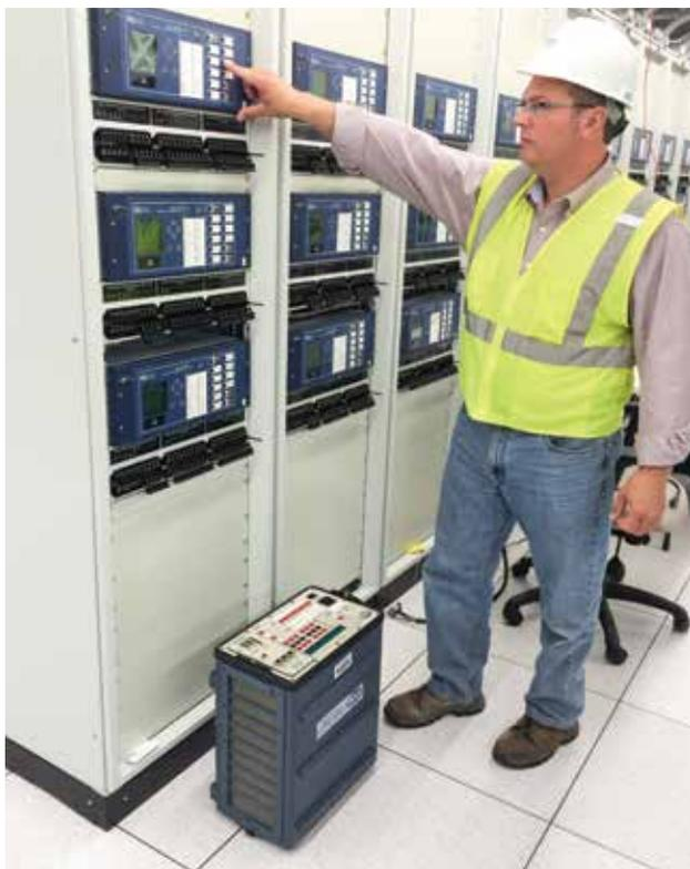
Kevin Mahoney testing the IEC-61850 based Advanced Protection and Control System (APCS) during 345 kV substation commissioning.
