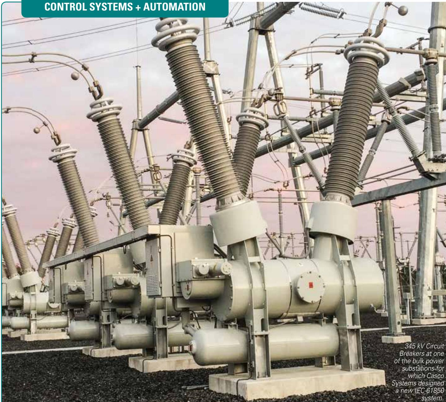
345 kV Circuit Breakers at one of the bulk power substations for which Casco Systems designed a new IEC-61850 system.
