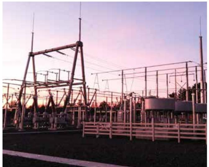
345 kV Substation Yard showing 'A' frame transmission line structure, circuit breakers and reactor bank.
